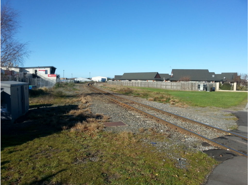
Kaiapoi: View looking southbound at potential station site
