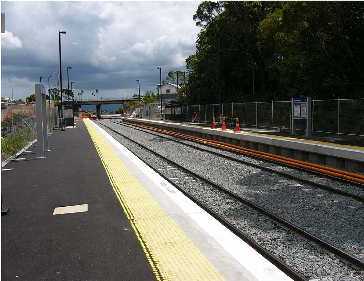
Example Temporary Platform (2 Years) Constructed at Avondale Station
