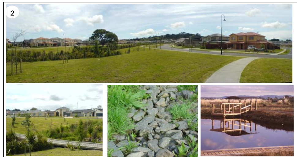
ABOVE FIG. 4-2: Examples of blue network responses that focus on improving local settings. These often result in increased levels of amenity and property value, greater surveillance and hence greater safety levels. Approaches that focus on slowing the movement of water also help reduce the risks of flash flooding and erosion / coastal degradation.
