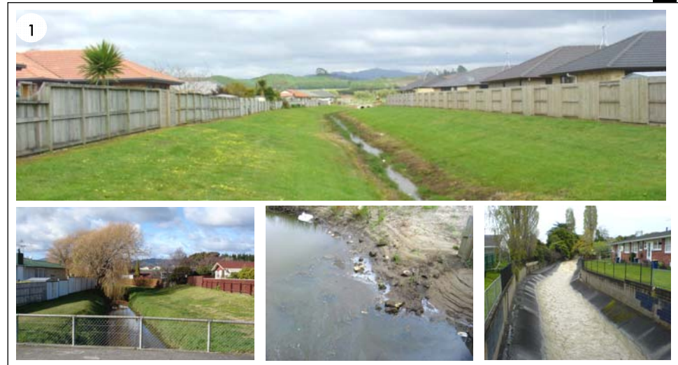
ABOVE FIG. 4-1: Examples of 'conventional' responses to blue network issues at the local level. These often poorly relate with their settings and create risks of flash flooding and result in the lowering of property values and safety levels.
